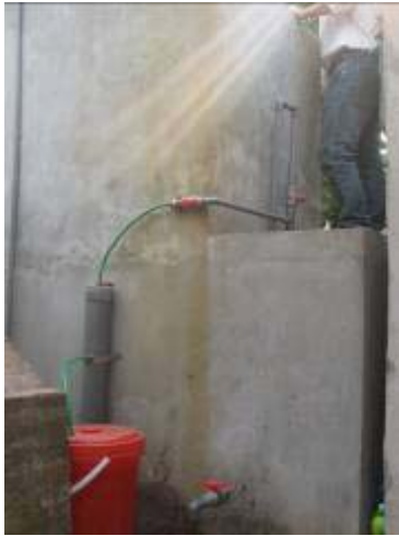
Some photos of the enhanced sand filter systems with GEH column for iron and arsenic removal with household scale in Mai Dong village, Hung Yen province.
