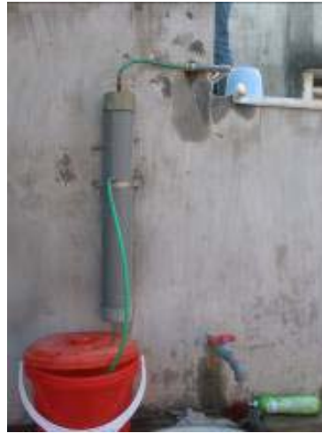
Some photos of the enhanced sand filter systems with GEH column for iron and arsenic removal with household scale in Mai Dong village, Hung Yen province.
